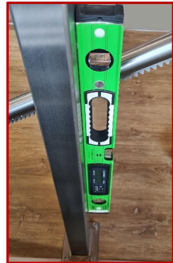
Figure 6: Aligning the columns
